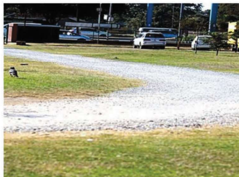
Photographic record — Driveway to Administration Block
